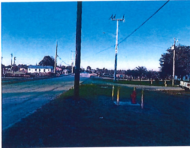
New pole recently installed.
